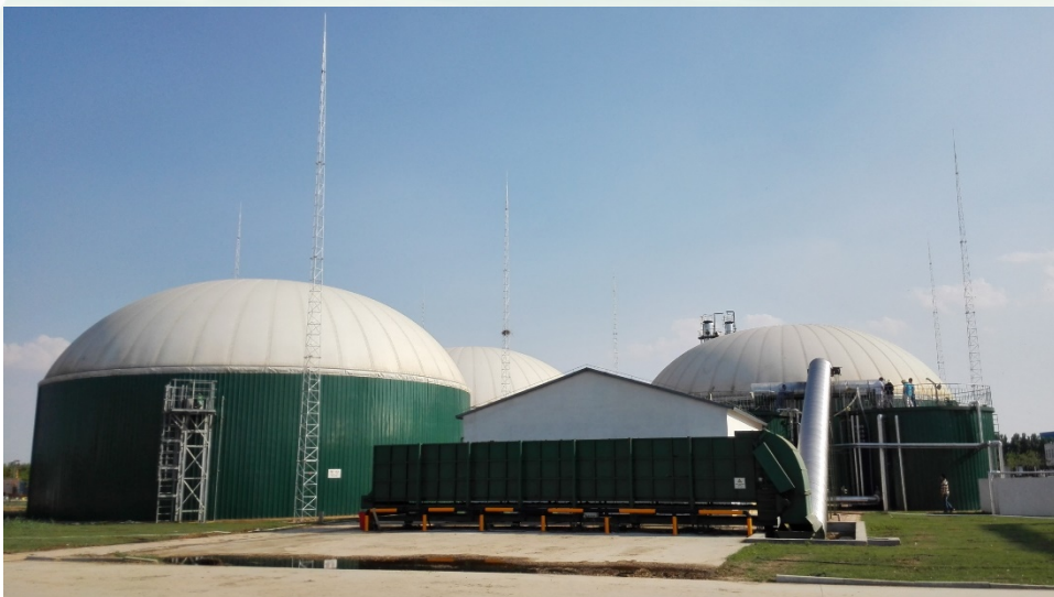
Corn/Wheat Straw Biogas Plant (CHP & CBG), China
